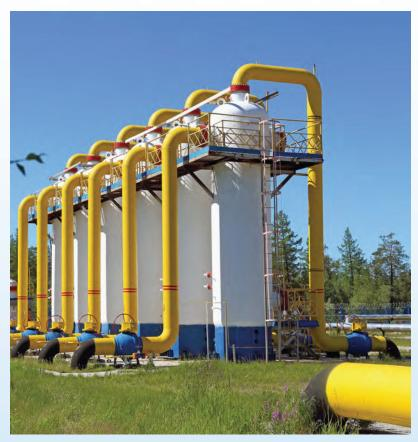
Removing siloxane is an important step in cleaning methane gases for use as fuel since siloxane is a form of crystalline silica that will essentially turn into glass when burned or combusted. The collection of combusted siloxanes inside of engine components can cause the buildup of heat, water, and other contaminants that can cause corrosion, leading to problems in the engine.
